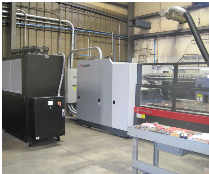
A 20-ton process chiller cooling a laser cutting system is built with a microchannel coil. The smaller coil reduces the size of the chiller and helps improve its energy efficiency.
